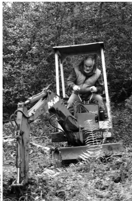
Jeff using his construction skills to build an artificial badger sett.
